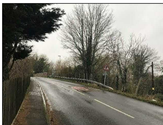
Figure 12 Main Road, approach to Appleford Station
