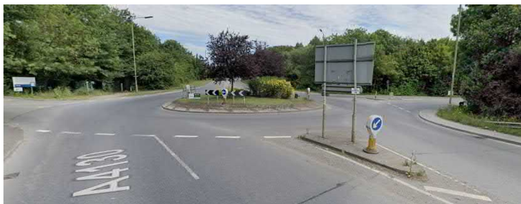
Figure 22: A4130, Purchas Rd and Hawksworth Roundabout
