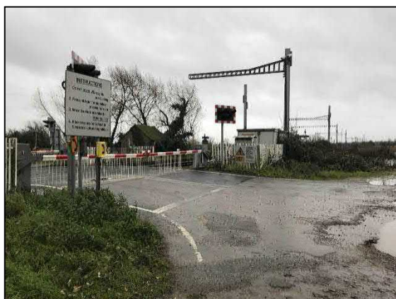
Figure 9 Appleford Level Crossing – west of railway line
