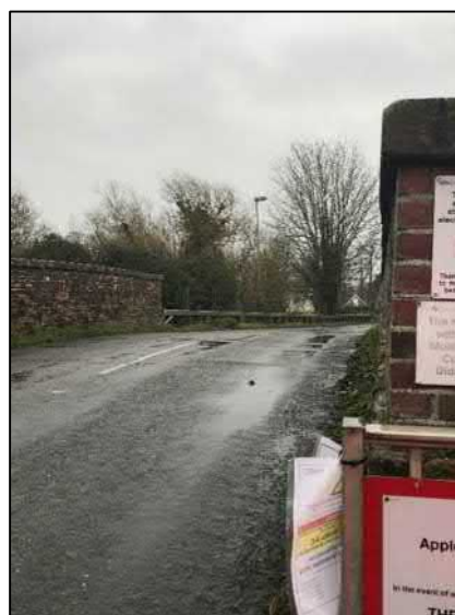
Figure 14 Appleford Station, western access – view to east
