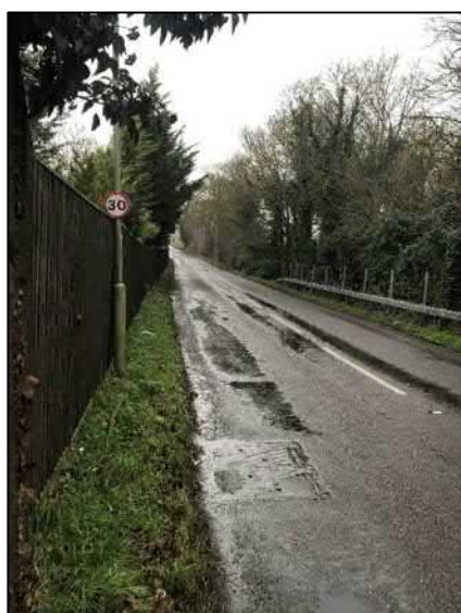
Figure 13 B4016, east of Appleford Station
