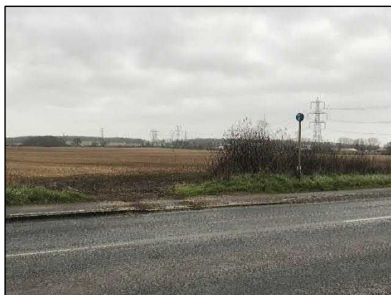
Figure 17 A415 Abingdon Road, shared use footways
